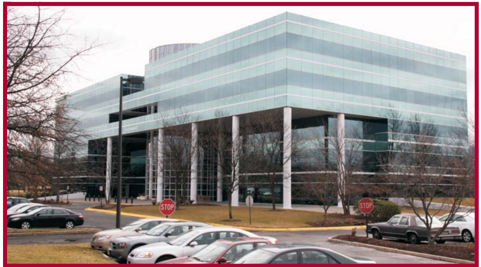
Atrium I, at 1000 Atrium Way, Mount Laurel, N.J., is AKCG's new base.
